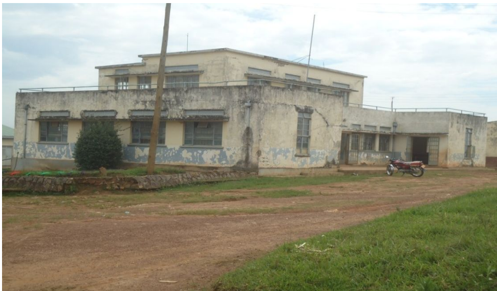
Picture 4.15: Old and Depleted Structures at KNRCC.
